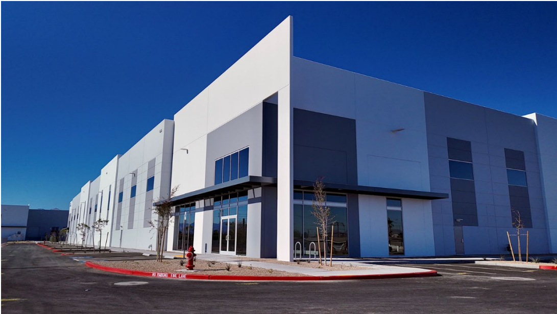
Picture: 2600 Carey Drive, Building D., North Las Vegas, NV- Wausau Coated Products New Facility
